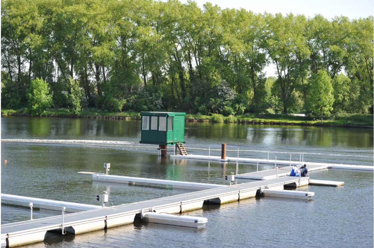
Hamburg Aligner's Hut
