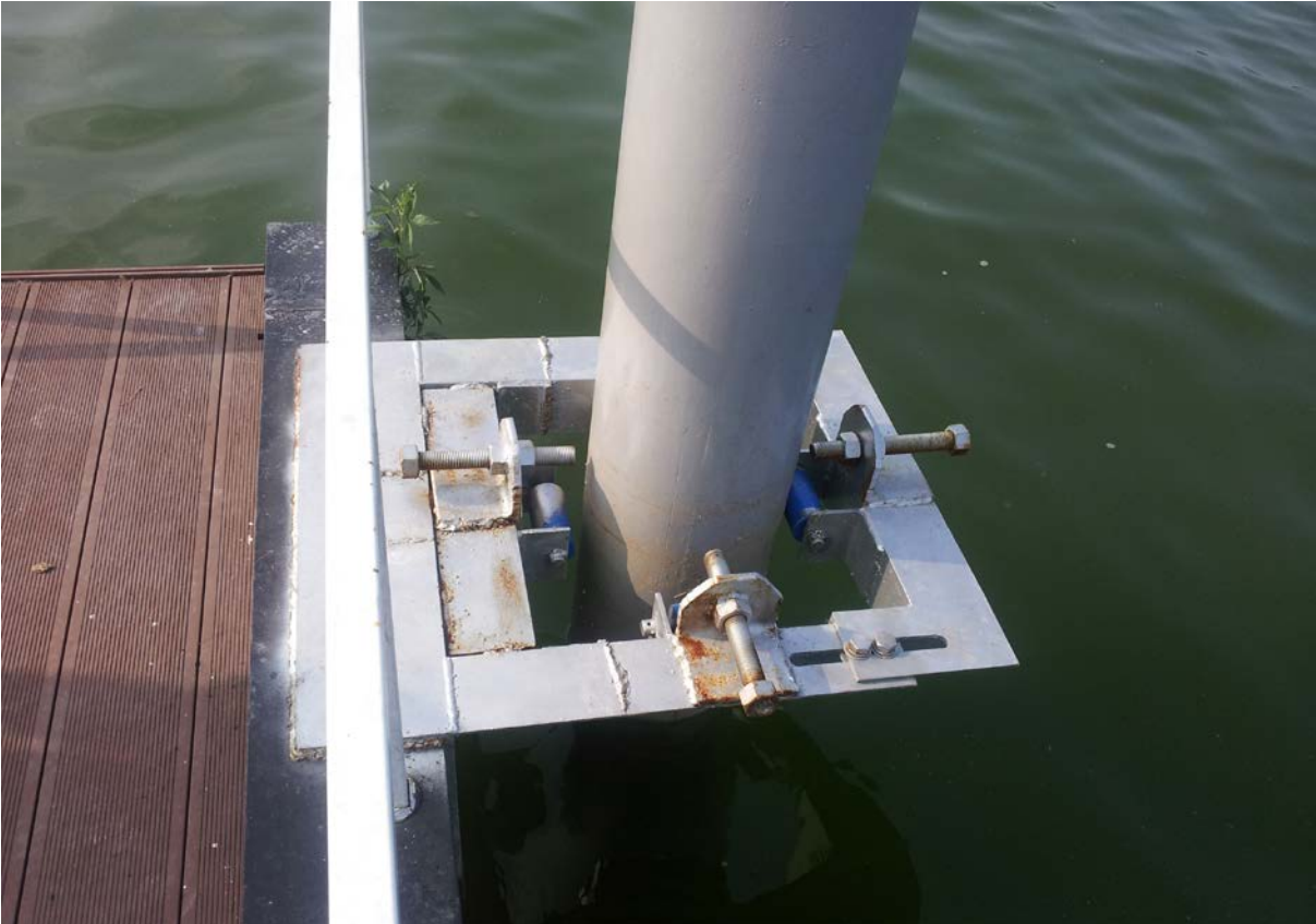
Floating Platform Fixing Chungju
