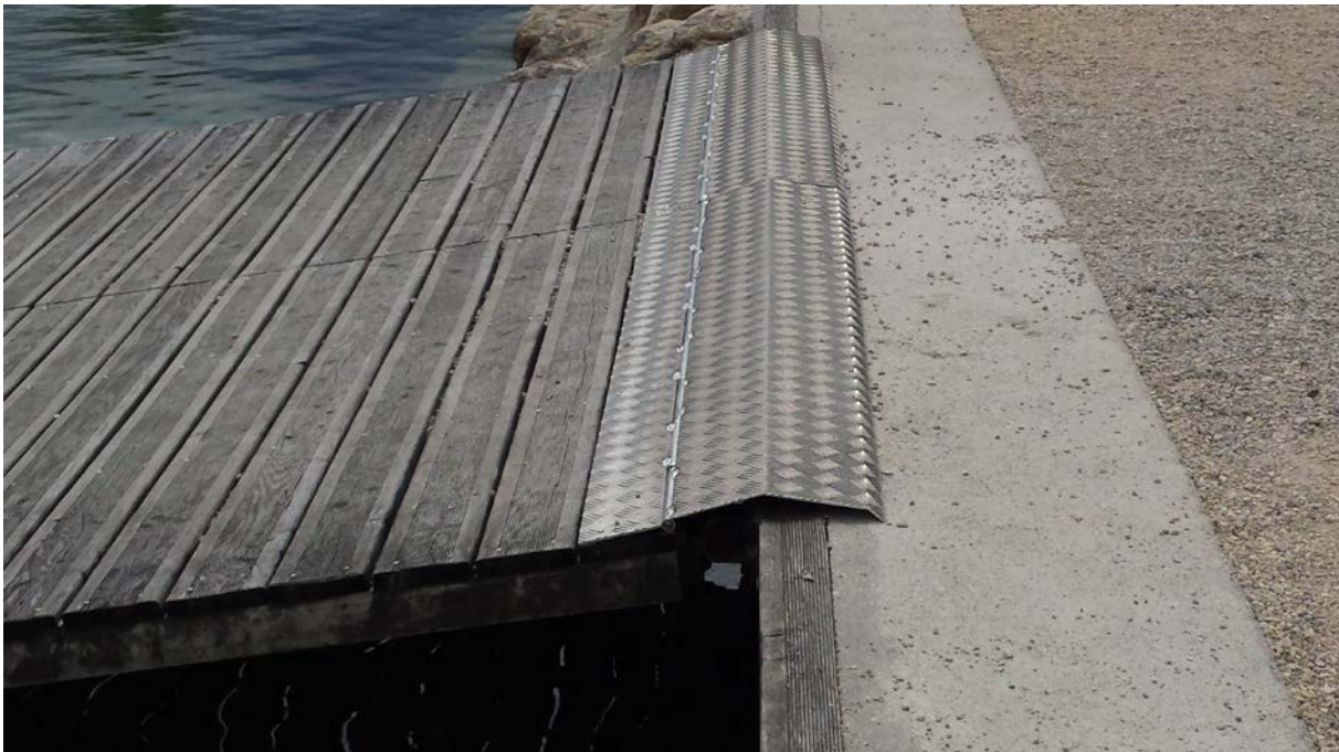
Launch Pontoons Fixing
