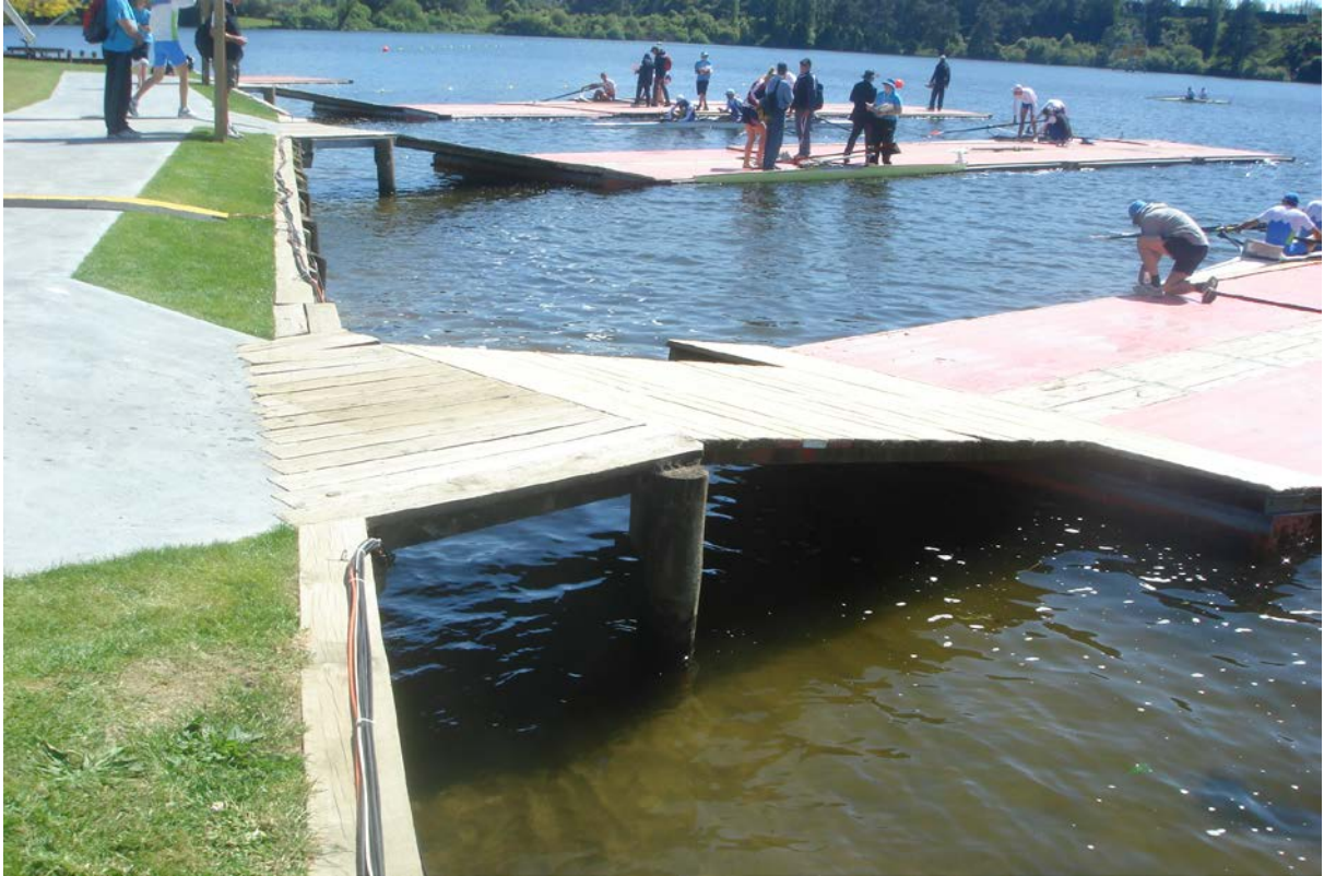
Launching Pontoon Fixing Karapiro
