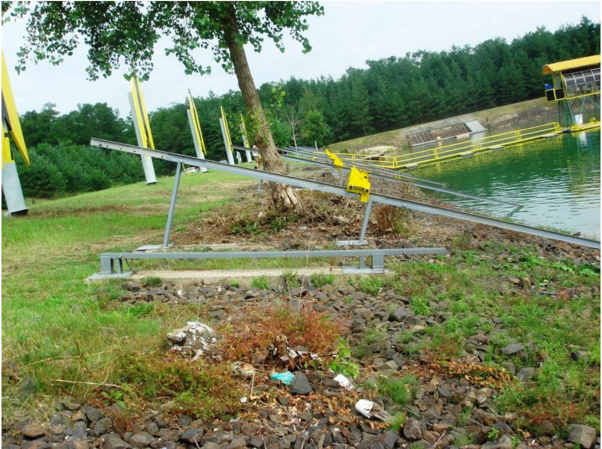
Anchoring Albano System Prague
