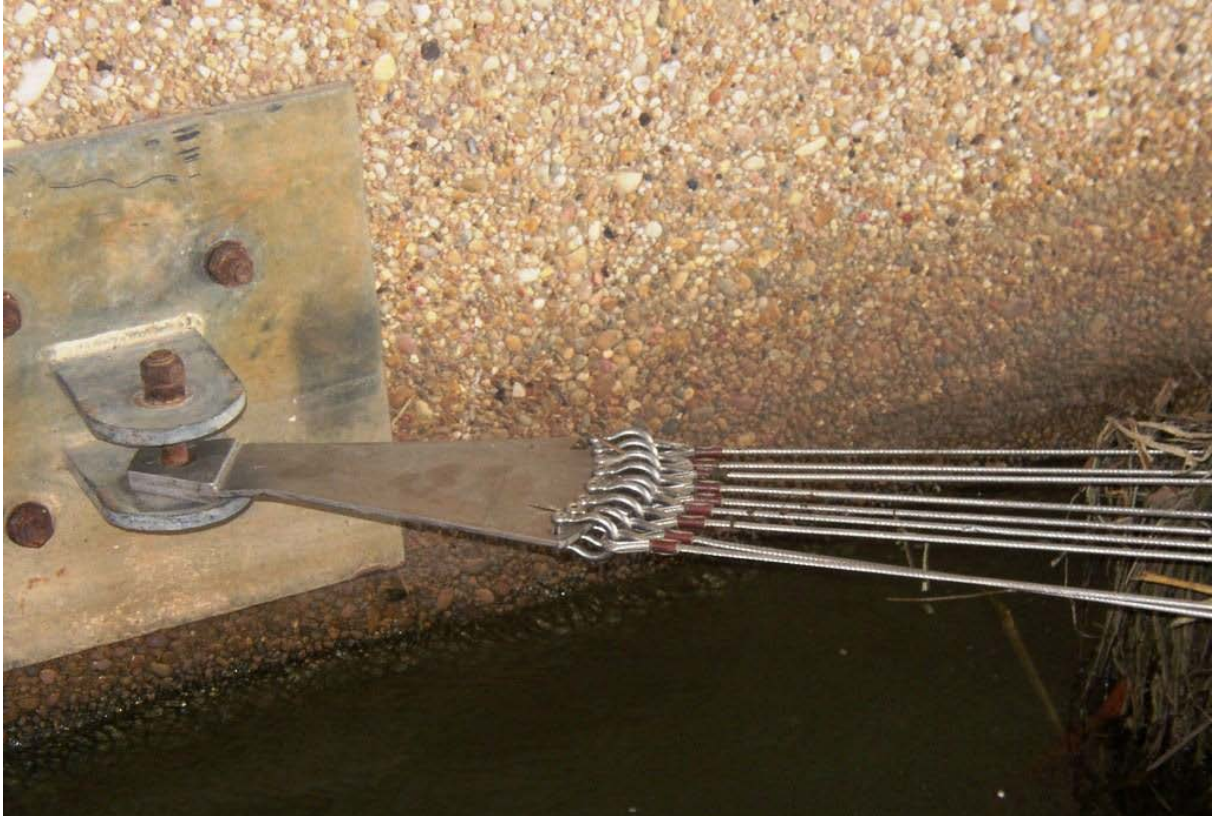
Anchors Albano wires Seville
